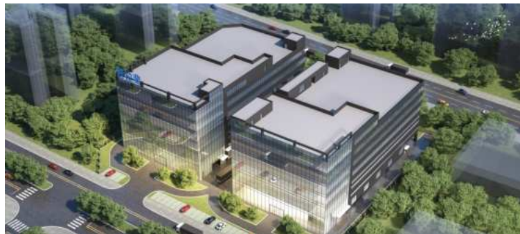
New Headquarter ( Running in July, 2025 )
